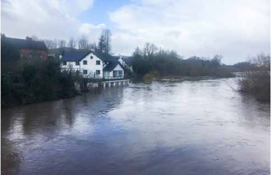
The River Teme floods a riverside home on the B4203 opposite Mill Farm Country Retail village, taken from the footbridge adjacent to Stanford Bridge (photo by Michael Whitefoot)
