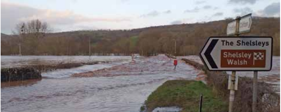
The River Teme waters surge across the B4204 access to Ham Bridge, taken from the Clifton-on-Teme side (photo by Jerry Johns)
