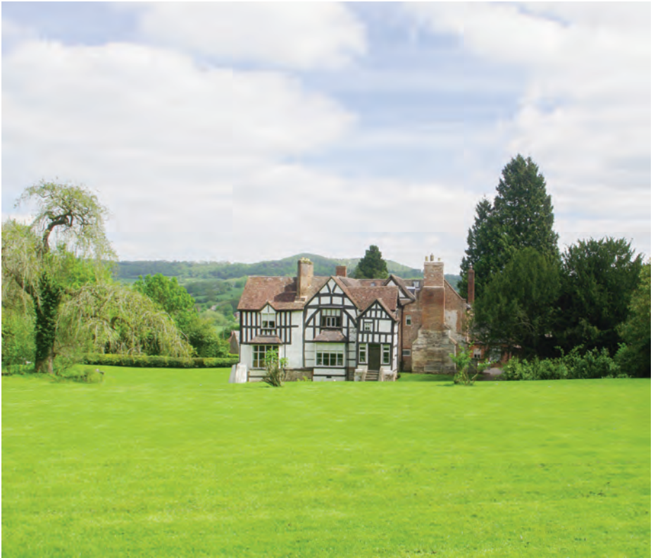
The Court House revealed
